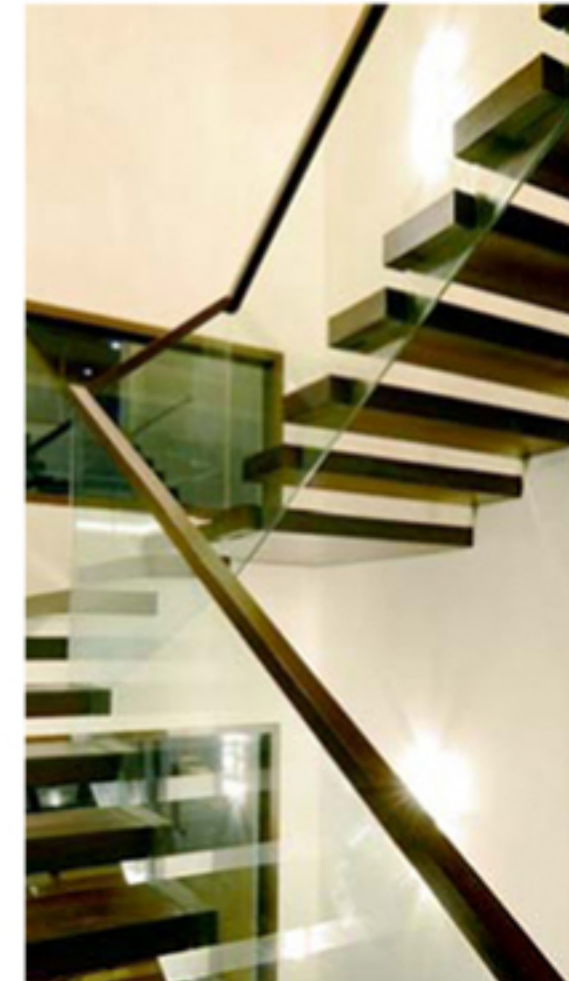
STAIRWAY: The reinforced cantilever staircase
